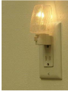
The outlets are live – note the lamp is lighted
